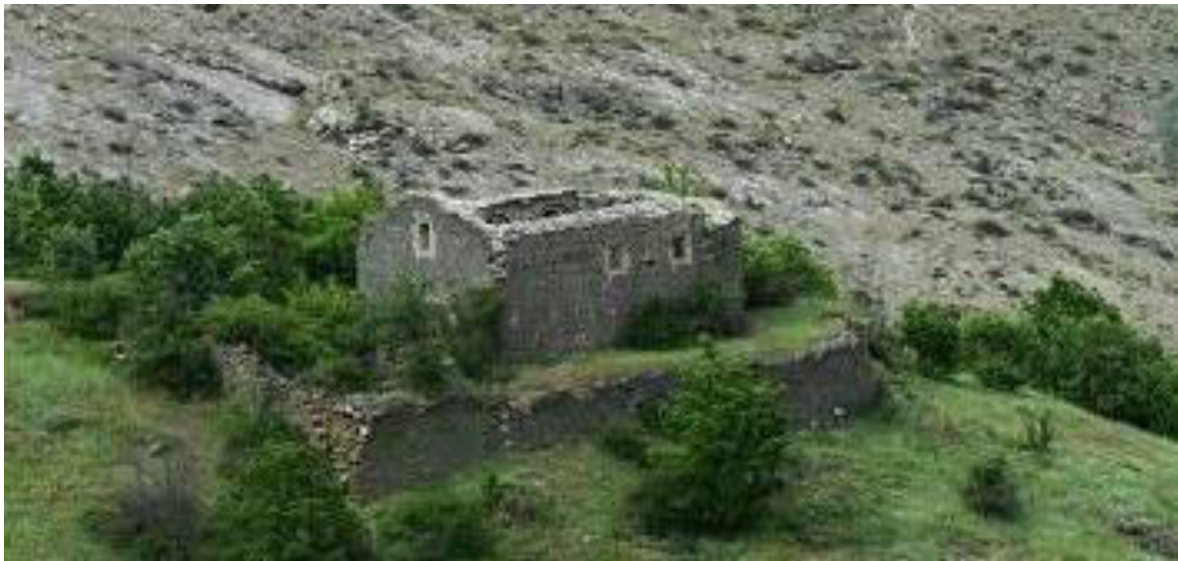
Plate 93: Vartli district church Güvemli village (name unknown, https://gumushane.ktb.gov.tr/TR-232434/torul-guvenli-koyu-vartli-mahallesi-kilise.html ).
