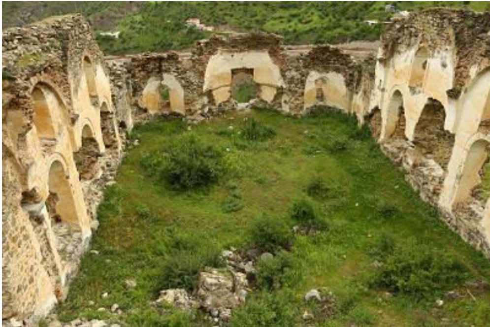
Plate 5: Inside the Surp Karabet Armenian church, old Gümüşhane ( https://gumushane.ktb.gov.tr/TR-231651/merkes-suleymaniye-mahallesi-surp-karabet-kilisesi.html ).
