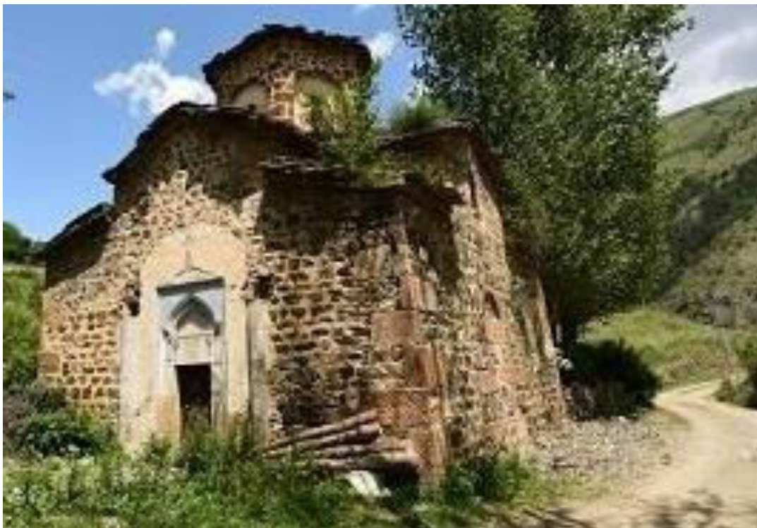
Plate 55: Alpullu (Greek Monobanton) Greek church, Stavri (name unknown, https://gumushane.ktb.gov.tr/TR-232440/torul-ugurtas-koyu-alpullu-mahallesi-kilise-1.html ).
